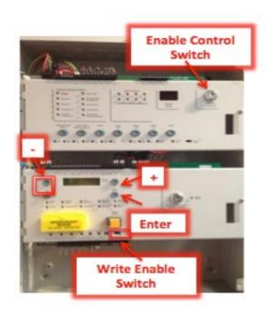
ALL OF THE FOLLOWING PROCESSES ARE CONDUCTED VIA THE EXTINGUISHING MODULES DISPLAY AND BUTTONS.
